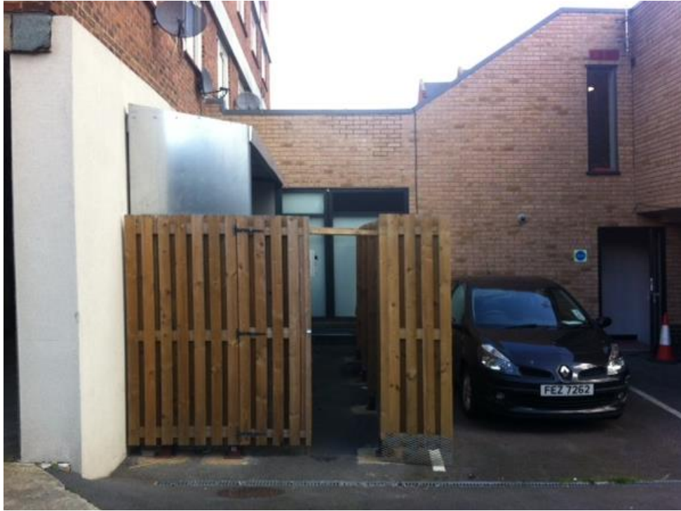
Image 2: Existing plant equipment including timber fenced enclosure
