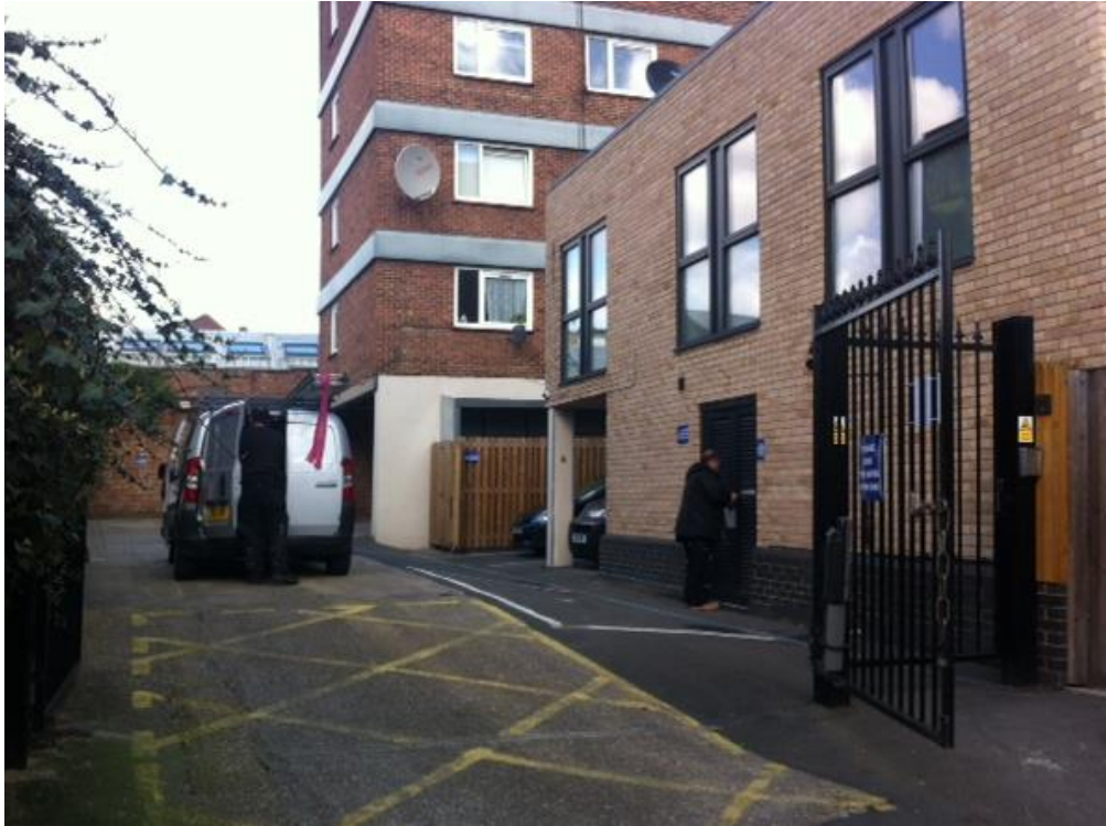
Image 4: View of plant enclosure from Mercers Road – timber enclosure to be replaced with black railings and louvre
